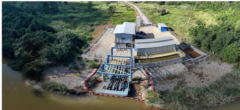
Water collection system in Valadares
