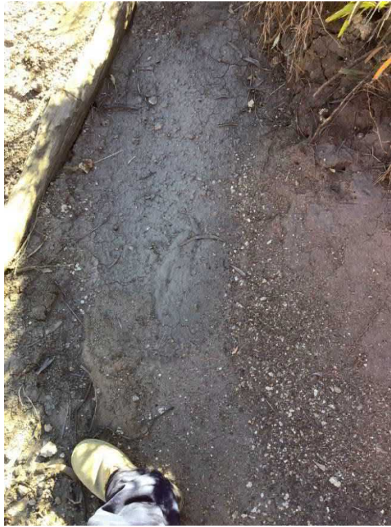
Photo 30 SW06 – Low Flow Channel
