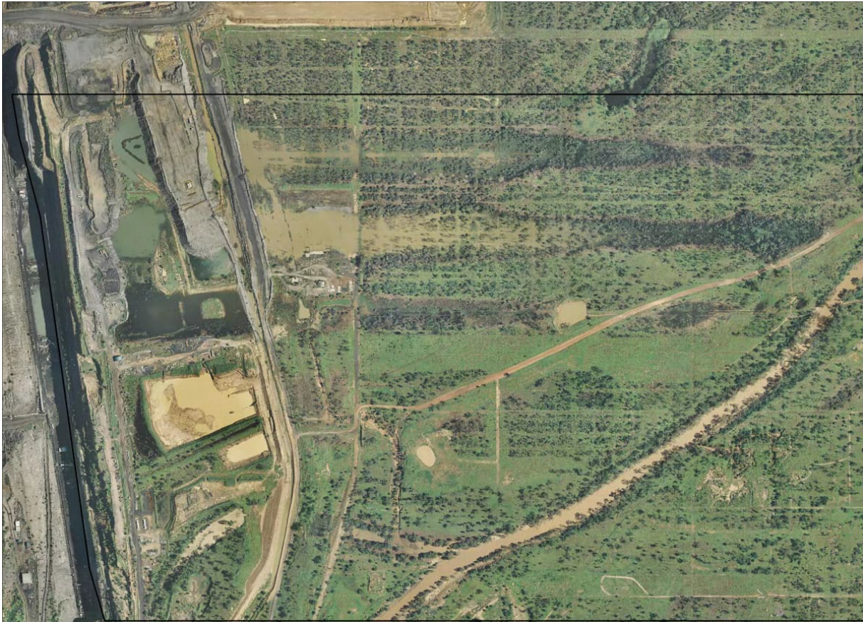
Plate 1 Flooded subsided longwall panels at the Bowen Basin Goonyella Broadmeadow Riverside Mine complex
