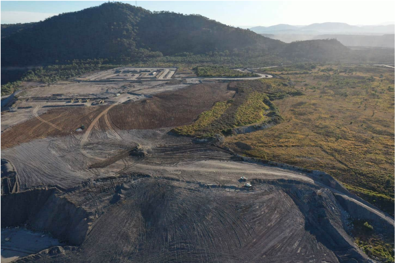
Figure 8 Bulk shaping and topsoil spreading at the Saddlers North emplacement
