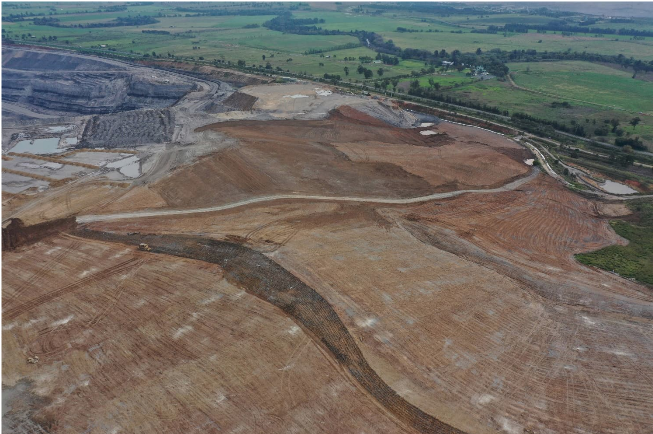
Figure 1 Rehabilitation works underway at VD5 along Denman Road.
