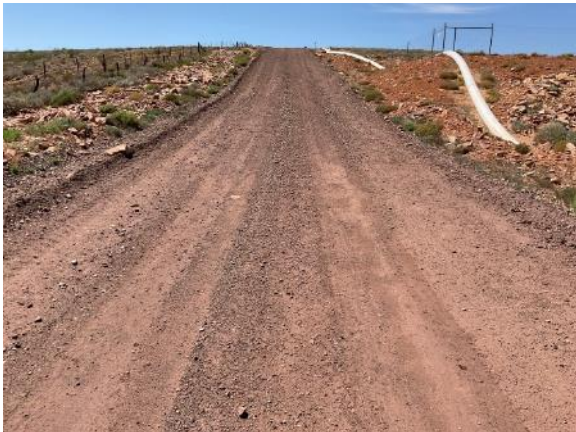
Appendix Plate A4.137: Facing east
