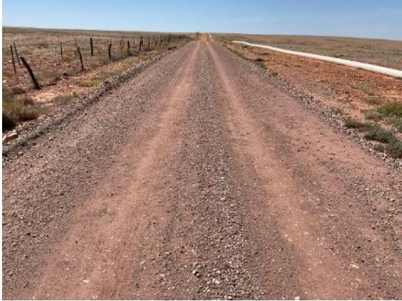
Appendix Plate A4.139: Facing east
