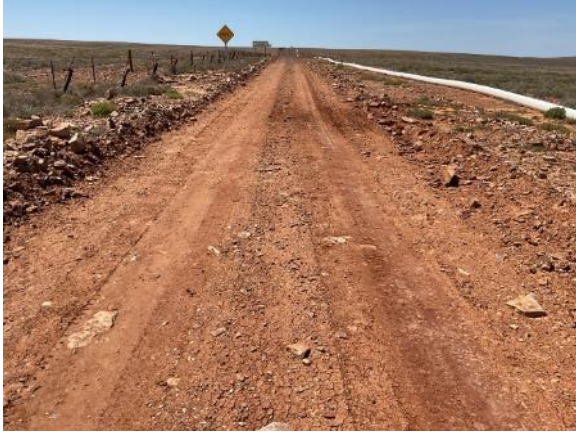
Appendix Plate A4.135: Facing east
