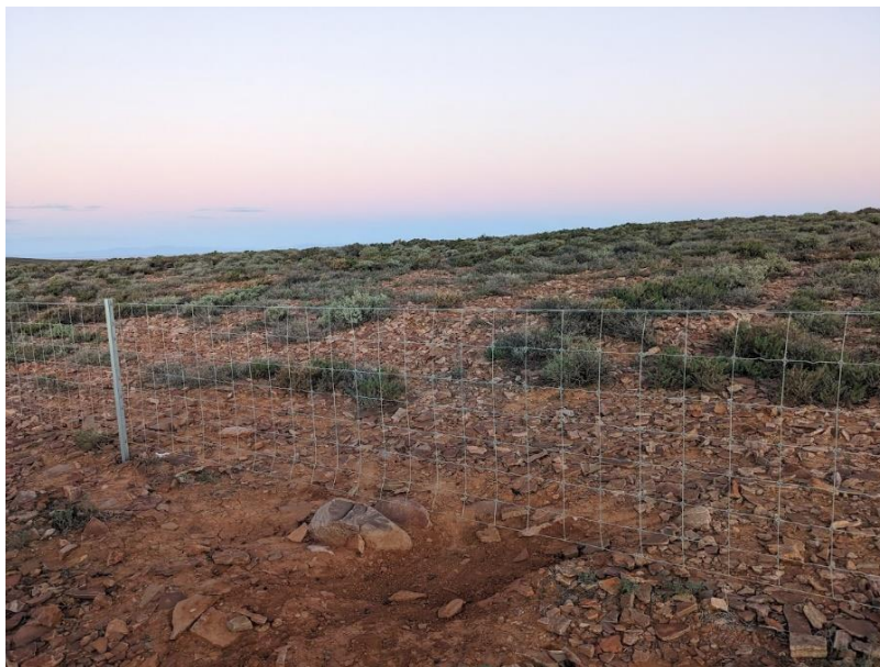
Figure 9. Example of a hole dug underneath the stock exclusion fence by kangaroos. These were patched up each time they were found with either large rocks or mesh wire.
