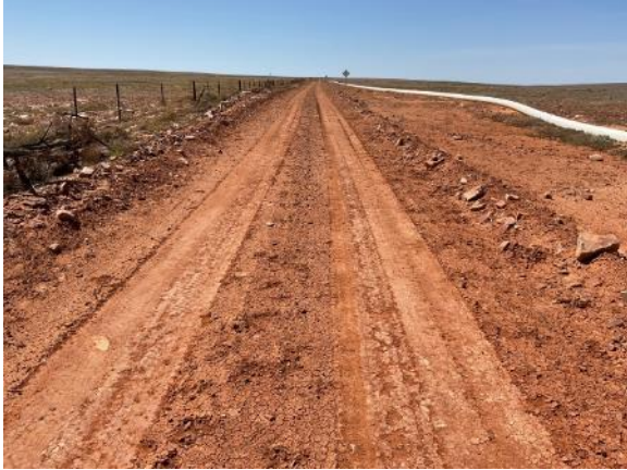
Appendix Plate A4.131: Facing east
