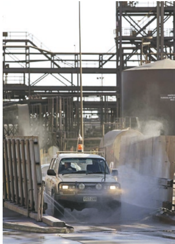
Plate 22.11 Vehicle wheel wash facility at the Olympic Dam gatehouse
