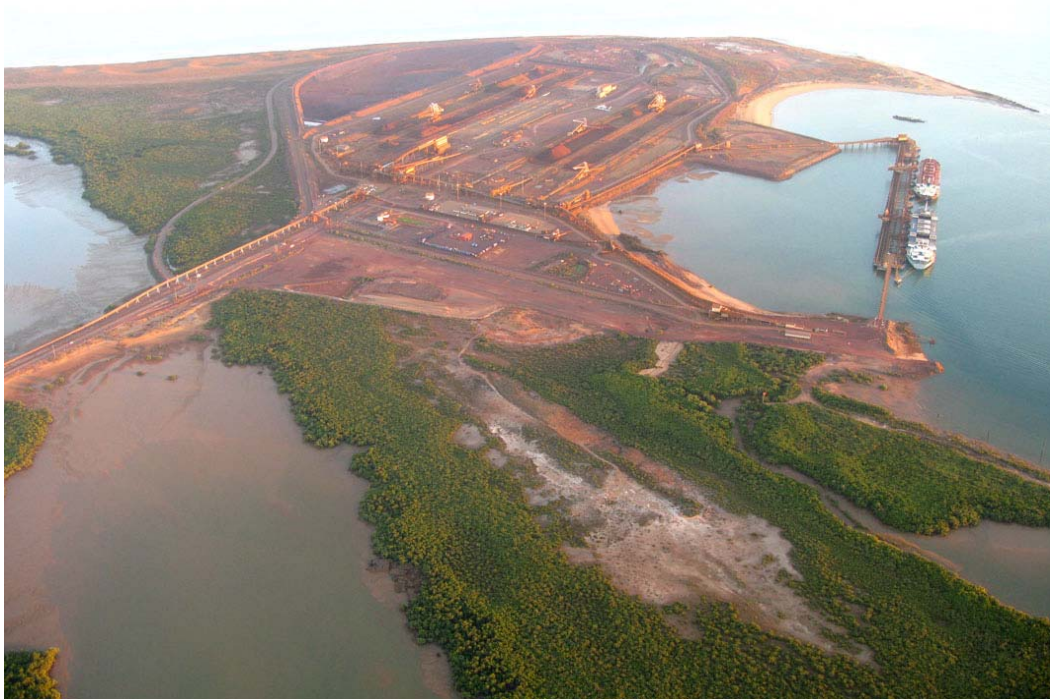
Plate 3.1. Finucane Island Loading Facilities in the Right Hand Side of Photo, Dunes Behind. Note the mangroves on Finucane Island in the foreground.
