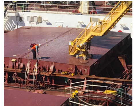
Figure 8: Access landed on hatch cover
