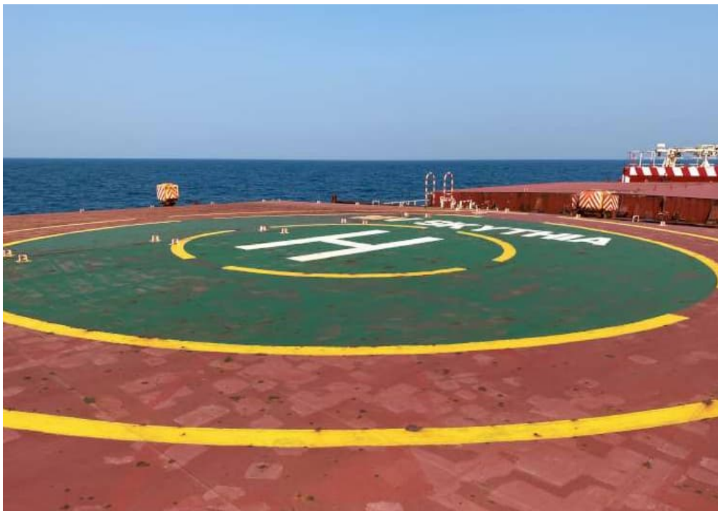
6. photos of the helicopter approach - please ensure the photos are taken from both port side and starboard side
